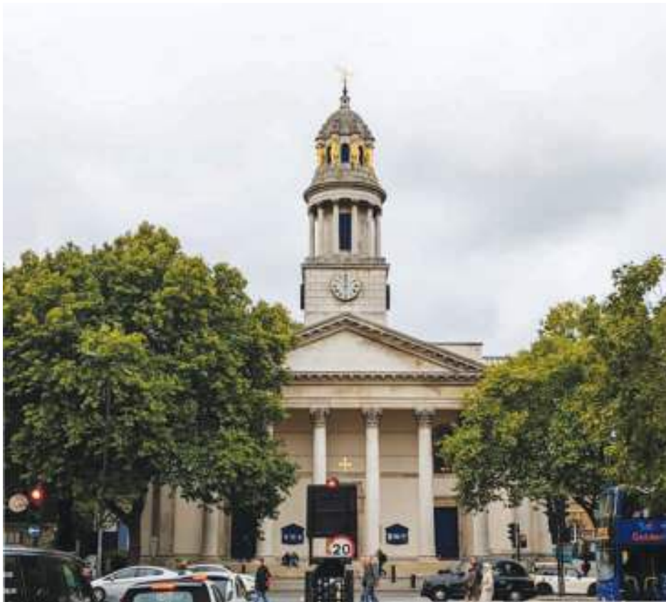
The church freed from its scaffolding.
