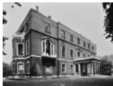
Bomb damage at Montagu House.
