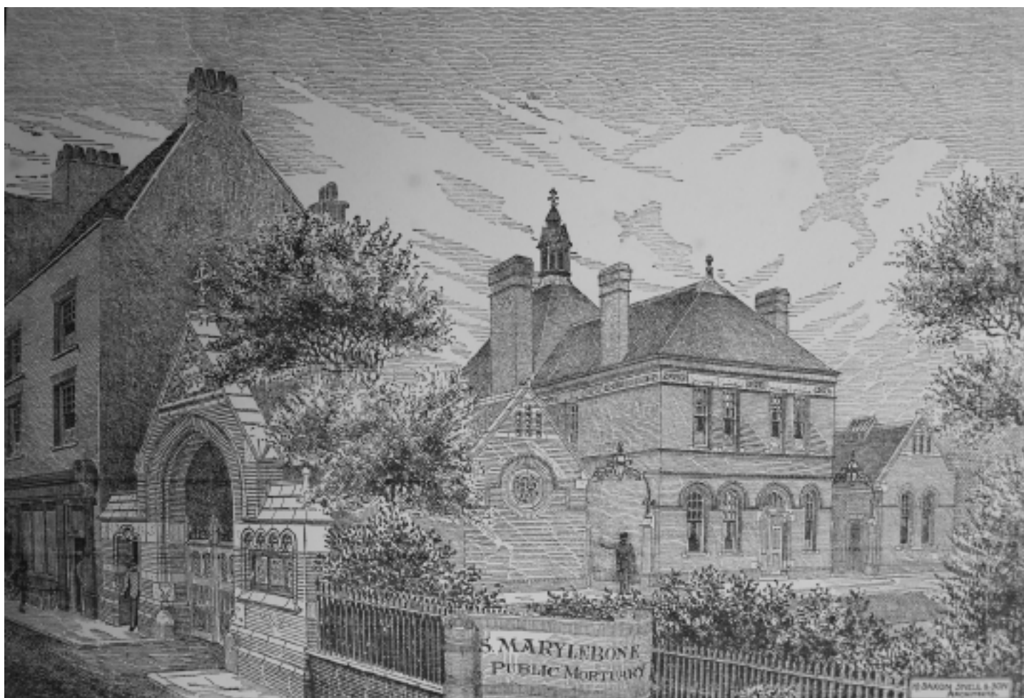
Fig 5. The new Mortuary and Coroner's Court with the gated entrance from Paddington Street. The left panel abuts No. 21 Paddington Street. Today, the right panel accommodates the plaque of 1981 commemorating Chateaubriand.
