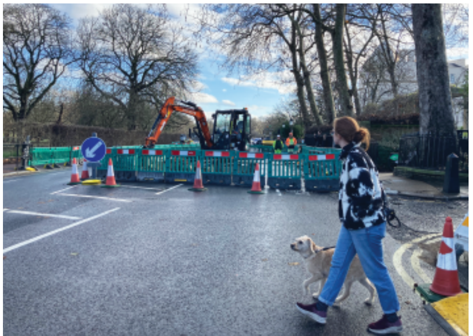
Work on the new crossing at Kent Passage.
