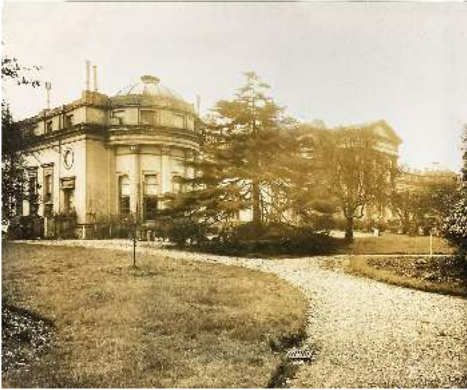
Fig.4. Exterior View of the west wing.
