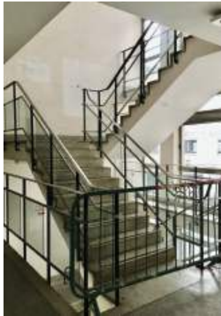
Original internal staircase and balustrade.
