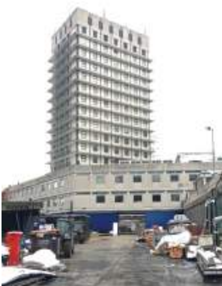
The 17-storey tower seen from an inner service yard.
